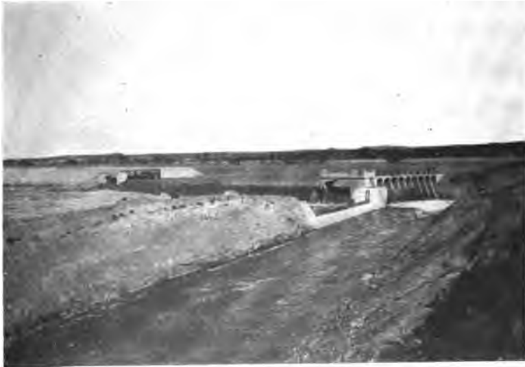
FIG. 95.—Whalen Diversion Dam and Headgates, Normal to Dam. North Platte River, Wyoming.
